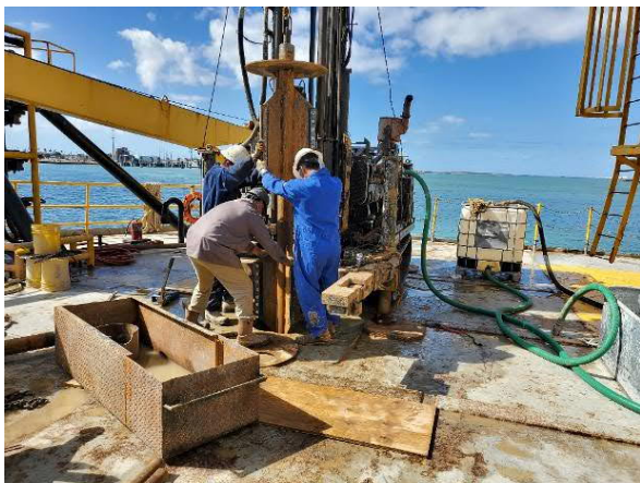
Photo 11 Advancement of boring CDP-08A utilizing drill rig equipped with direct-push technology.
